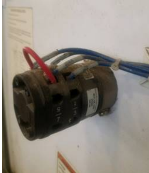
Image 1: The red wire demonstrates the ease of defeating a control circuit interlock.
